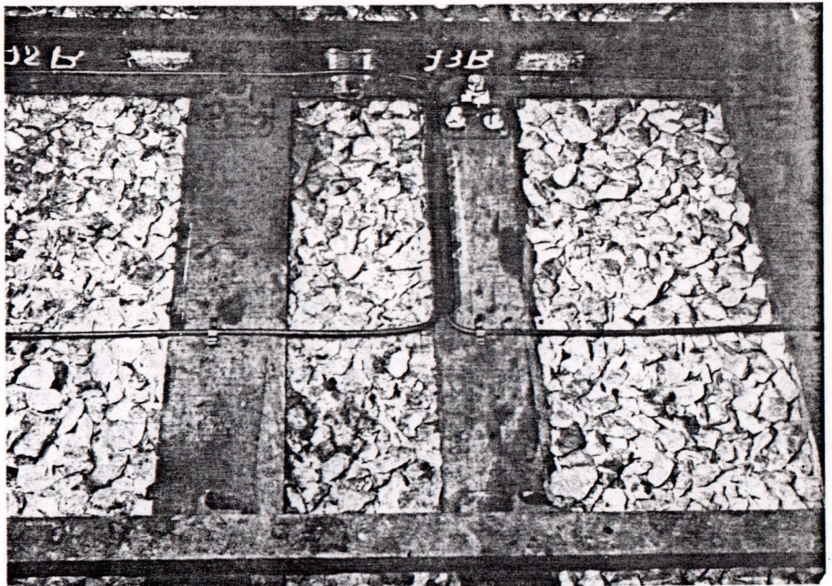
7. Transmissiekabel spoor-machine.
